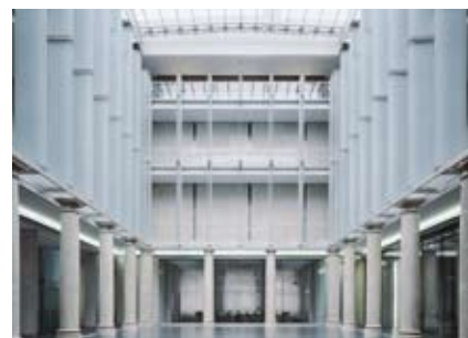
Former bank of the „Free State of Bavaria“
