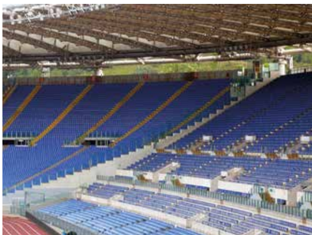
Fig. 3 The new insertion in the Olympic Stadium; the difference between the old and the new part is visible
