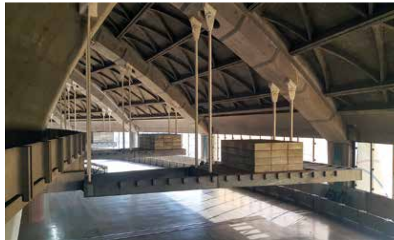
Fig. 4 Interior view of the Stadium circulations showing the innovative structural system of prefabricated-concrete cantilevered consoles
