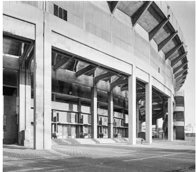
Fig. 9 The reinforced concrete extension ring around the oval stadium core (1992)
