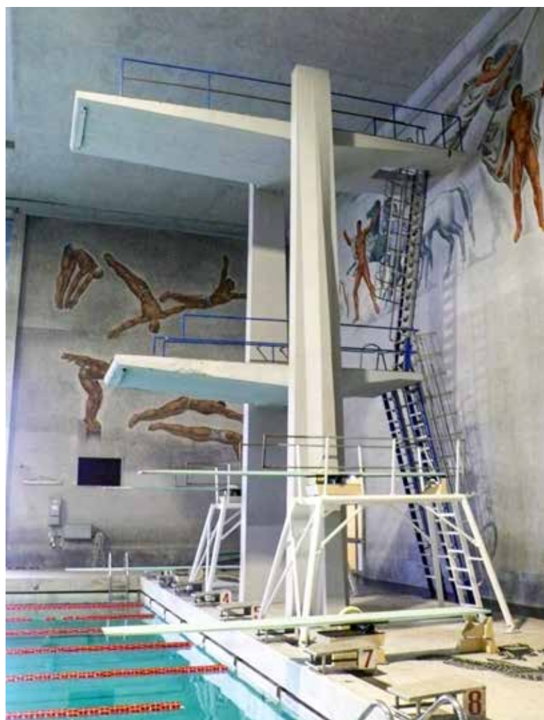
Fig. 4 The interior of the “Stadio del Nuoto”: the swimming pool with additions made by P. L. Nervi
