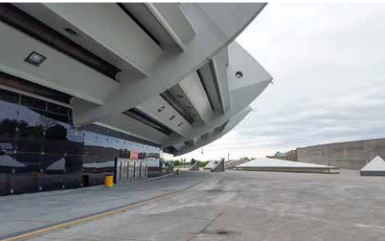
Fig. 3 The junction between the Stadium and esplanade showing the console structural system, its expressive use of concrete and original glass wall
