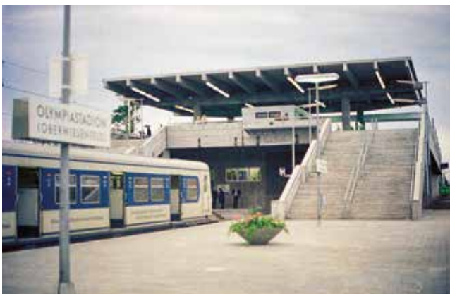
Fig. 1 Railway station building shortly after opening
