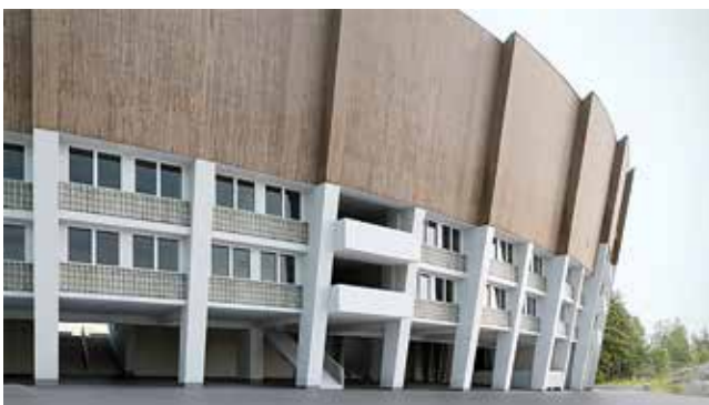
Fig. 6 The Olympic facade after its conversion, 2019; the new exit staircase 3rd bay
