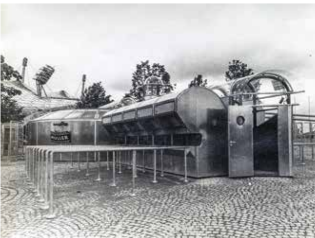
Fig. 6 Ticket booths SO1 at the south entrance of the stadium (PAS Archiv)
