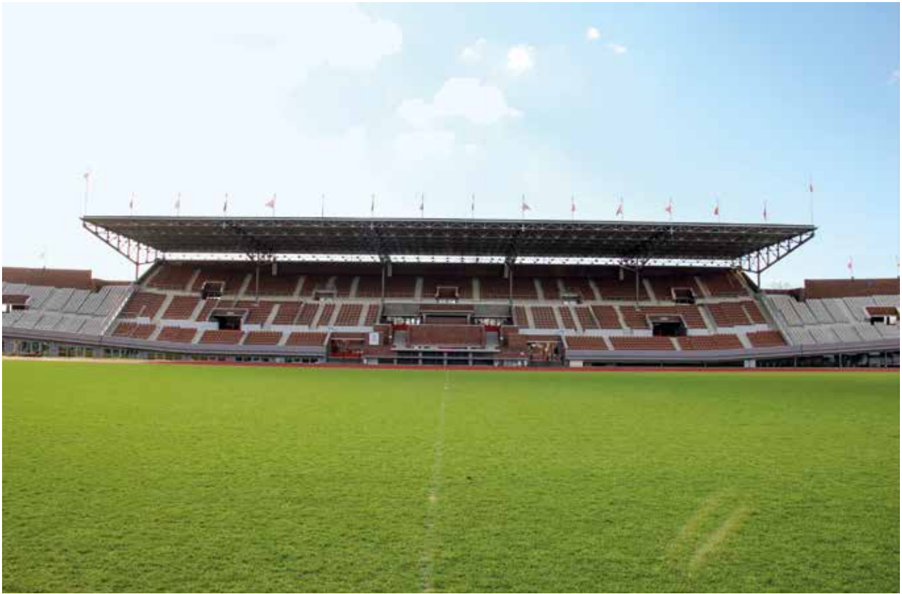
Fig. 11 The Olympic Stadium, view of the west wing after restoration (2019)
