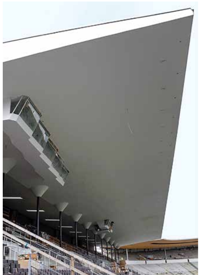
Fig. 7 The preserved western grandstand
