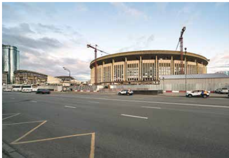
Fig. 5 Olympiysky Sports Complex and Swimming Pool during conversion/demolition
