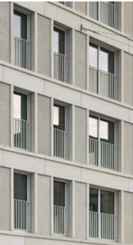
1 Fassadenfelder in Grobputz
